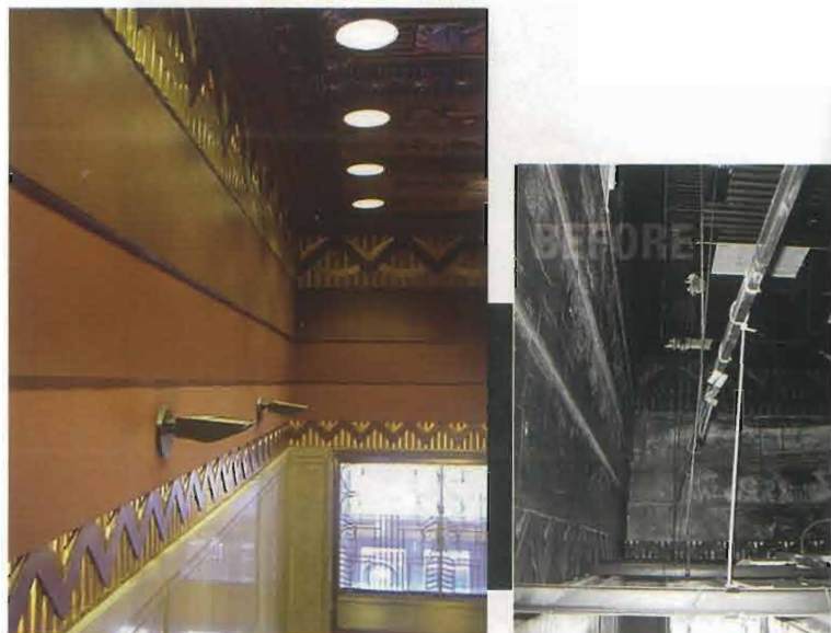
The Northcourt Building, recognized as a building of historical significance, had been damaged by a fire in the 1950s. Restoration revived the dramatic, open lobby and the original multicolor decorative plaster ceiling.
